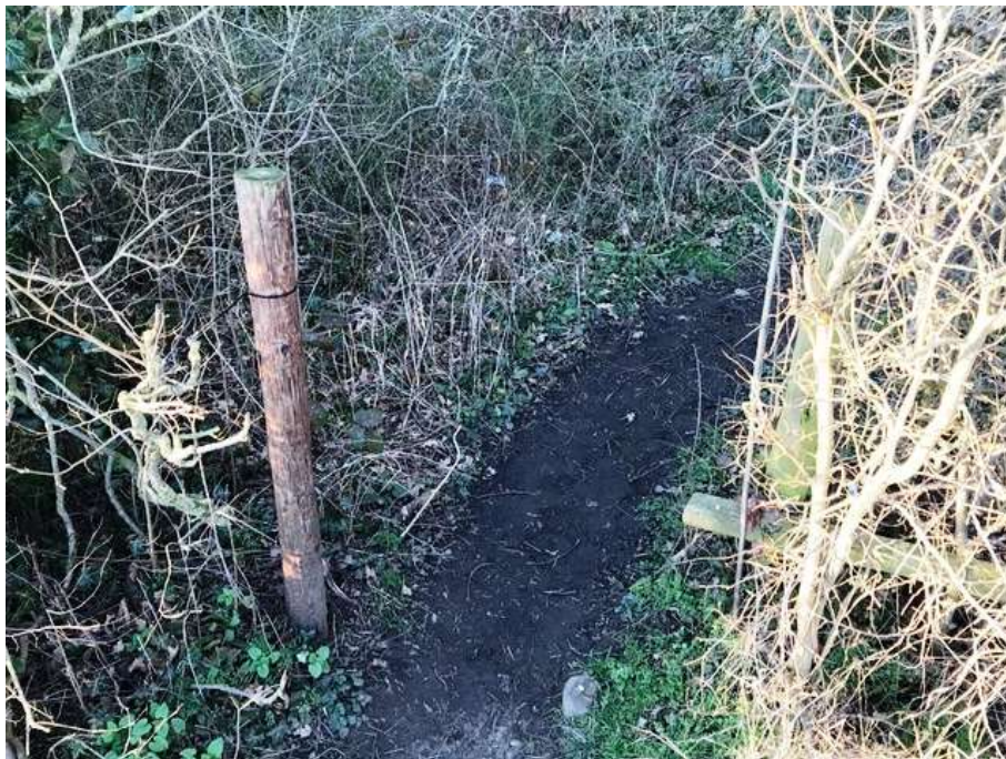
Photo B: Gap in Fence
